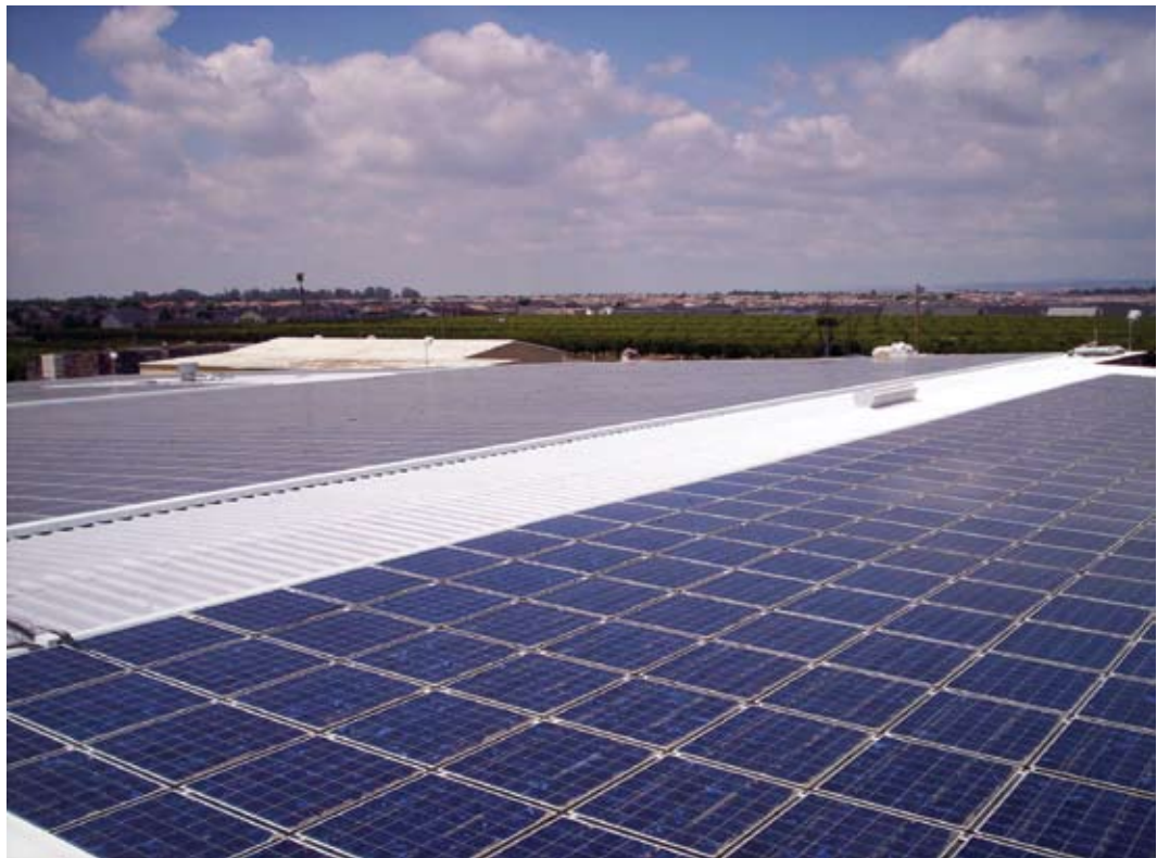
P-R Farms in California's San Joaquin Valley uses the electricity created from a photovoltaic system to power its cold storage and packing operations, resulting in a dramatic reduction in monthly energy bills. Credit: PowerLight
