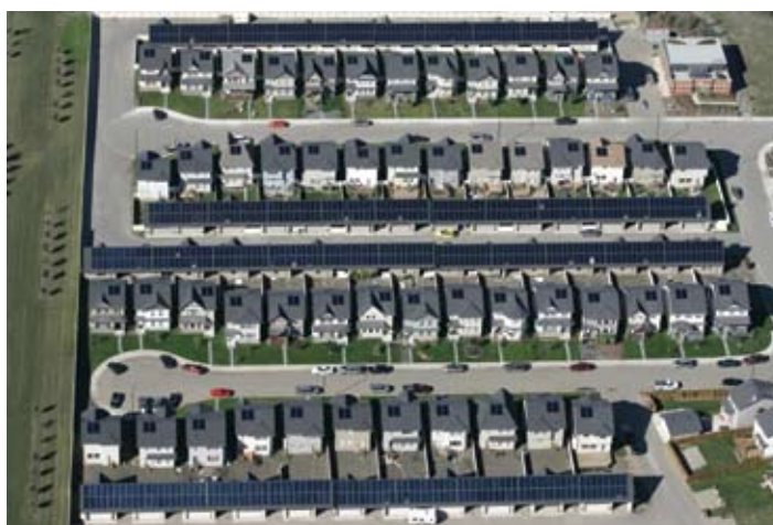
Solar energy can power communities across the nation, even in northern climates. The Drake Landing solar community in Okotoks, Alberta, Canada, just south of Calgary, relies on the sun for 90 percent of its space heating needs through the use of a solar district heating system with seasonal storage. Credit: Natural Resources Canada
