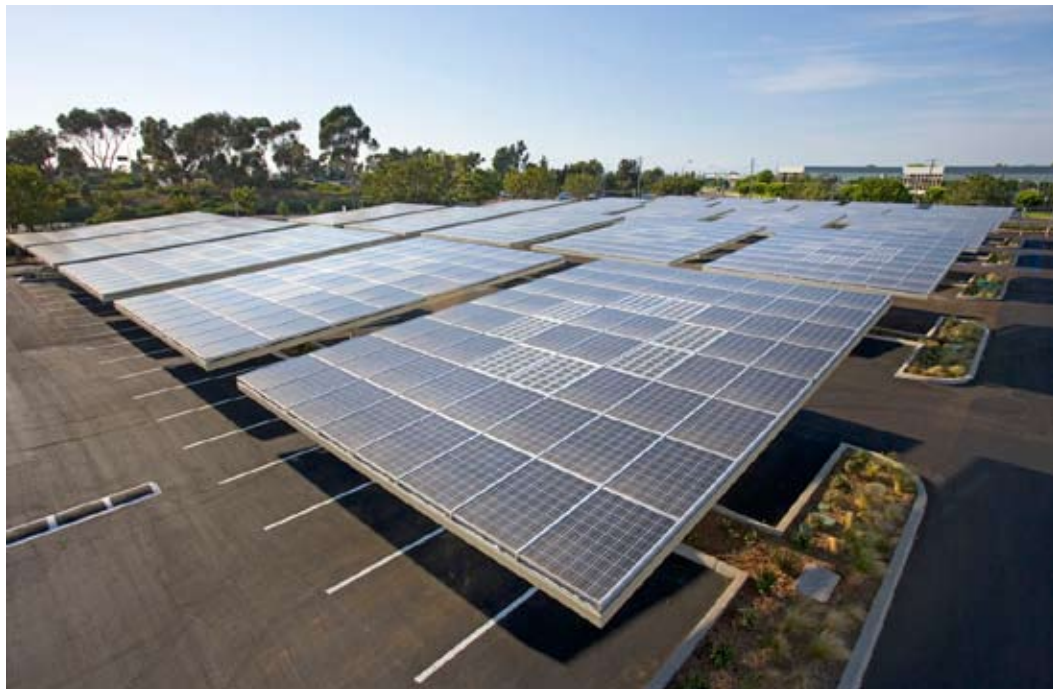
America has tremendous potential to capture energy from the sunlight that strikes rooftops and paved areas, such as this parking lot in San Diego. Credit: Envision Solar
